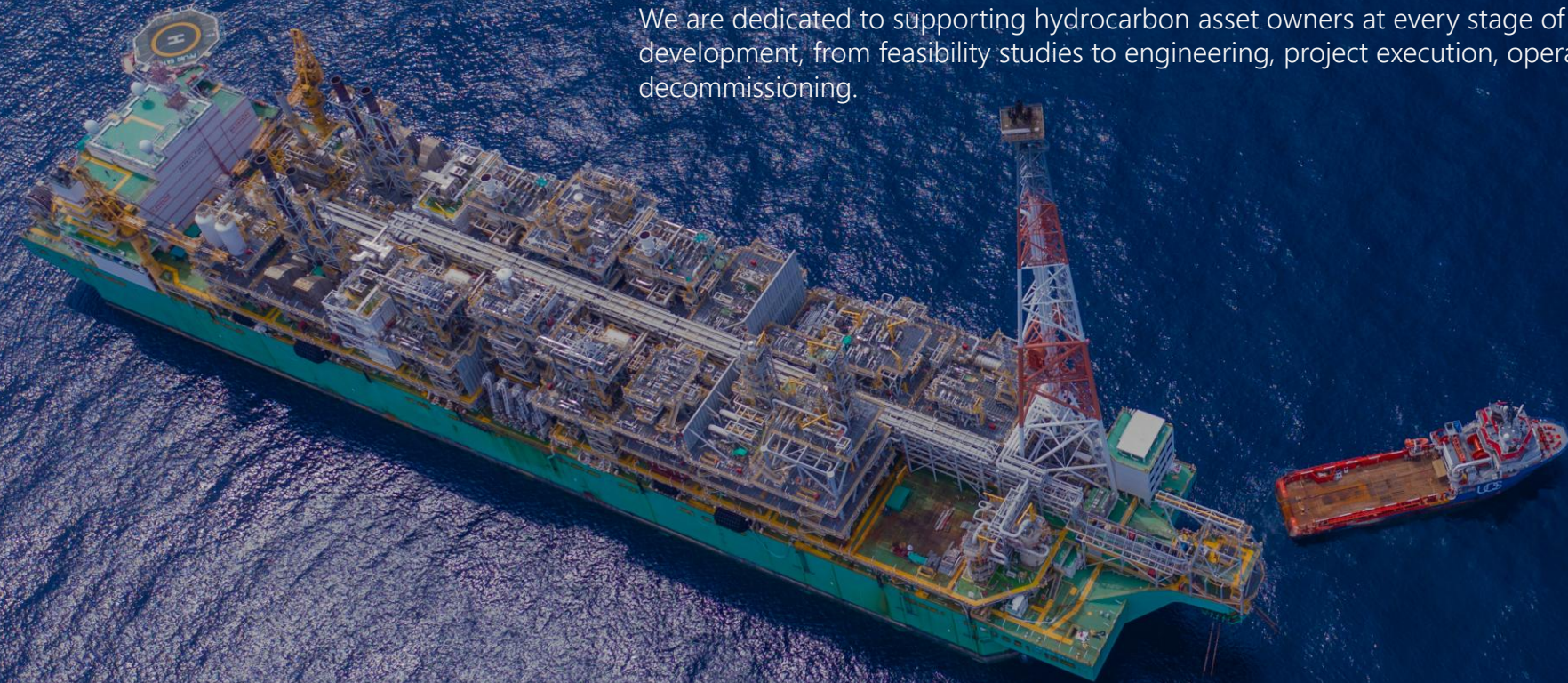
Photo from: Transportation & Installation of PFLNG Satu Relocation Project, Year 2019.
